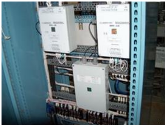
Figure 5. LIRA device in a 110 kV substation
