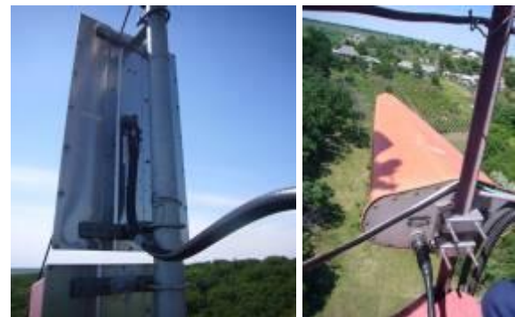
Figure 3. External appearance of the antennas: TVA 31/50 and TVA 51/50 (from the left); LAP 4/5-50/16 (from the right)
