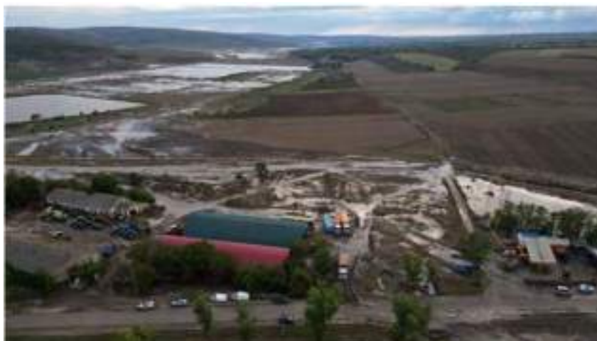
Figure 3. Property, land affected by heavy rains
