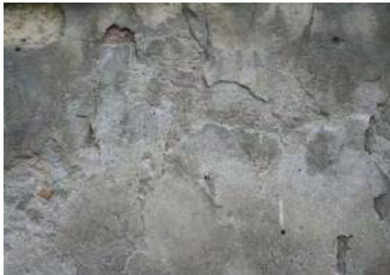
Figure 2. Chemical Degradation [2]
