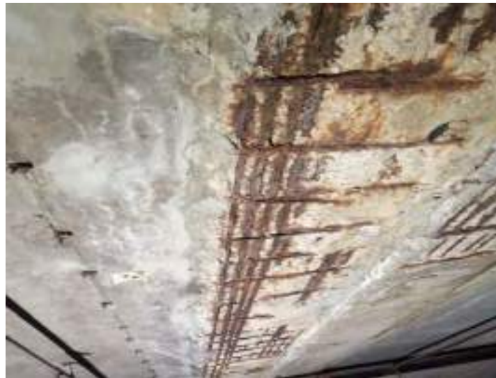
Figure 1. Rebar corrosion [2]
